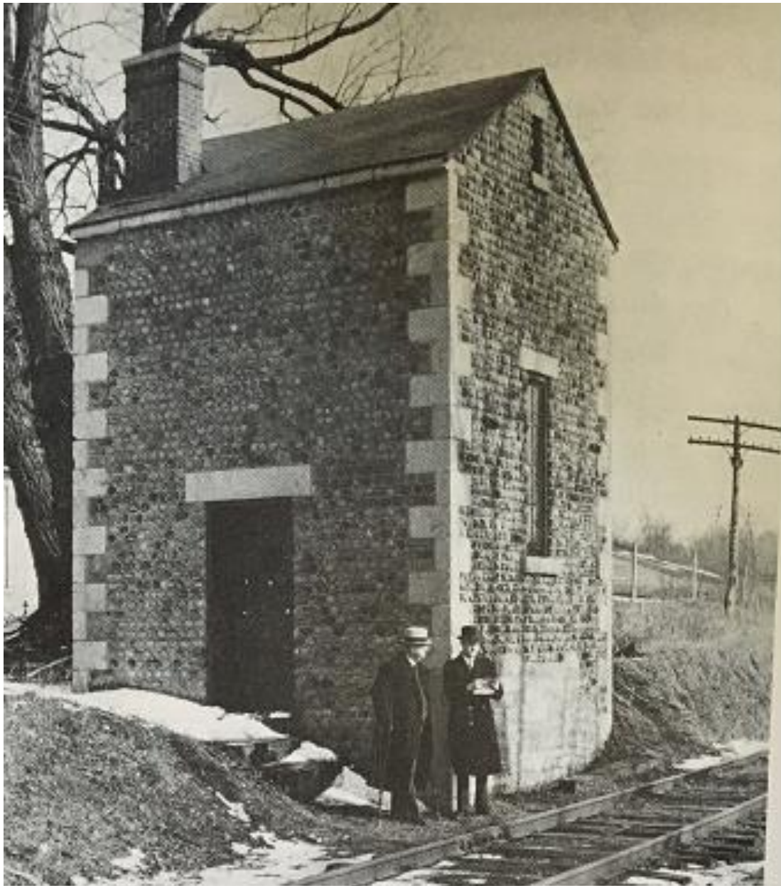
The 1845 Cobblestone Pump House at Fishers. ward Hungerford, Vice-president of the New York Central ilroad and noted railroad historian, who helped save the building in 1937, and J. Sheldon Fisher, Victor Historian.
